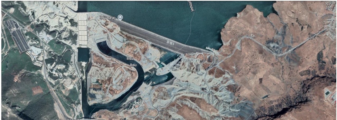
Figure 1. Ilisu Dam (Source: Google Earth, accessed on Jun 15, 2025)
